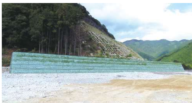
落石・雪崩・崩壊土砂防護補強土壁
